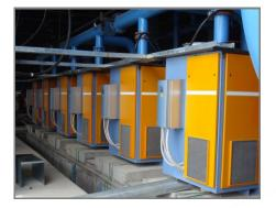
The systematic replacement of water cooled pumps with Pneumofore UV50 units at HNG involved in 2012 the Naidupeta and Nashik plants, where a new logic was installed, combined with a Variable Speed drive and an Eternet card for each vacuum pump.
