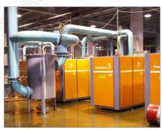
fluctuations of vacuum capacity. Thus, there is always just one pump running off the highest efficiency point, using the Variable Speed. All pumps happen to be the Master, as they follow together a simple logic of sequence, so that finally all machines have the same load and working hours.
